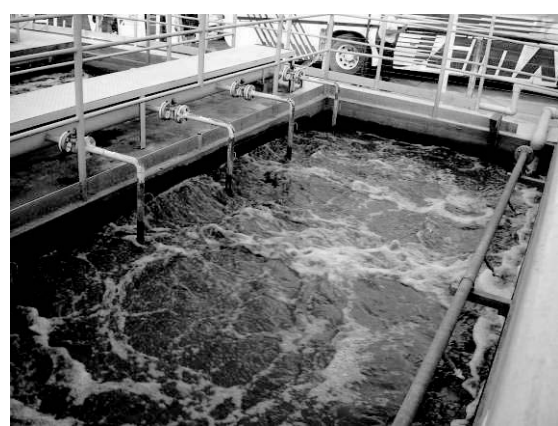
A water treatment facility at a PIM factory. There is no wastewater treatment facility in Manaus, so factories must treat industrial effluent as well as domestic (non-industrial) wastewater themselves.
